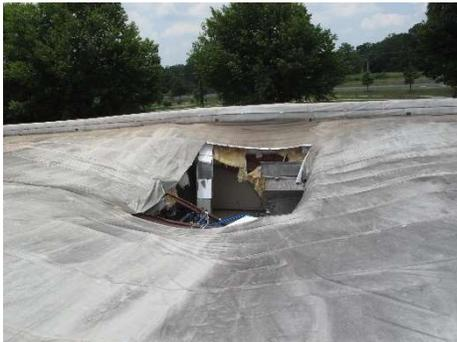
4. Is there an existing parapet gutter or valley gutter they are planning to fill with foam? If so remember it is NEVER acceptable to allow water to pond or stack on the roof, even for a short period of time. Several building collapses have been caused by this in recent years.
